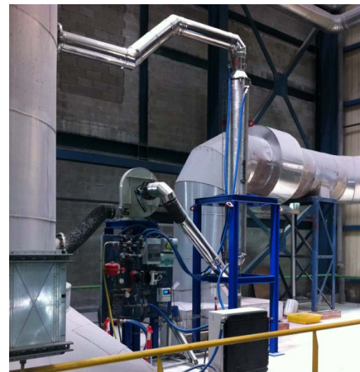
Waste to Energy Plant: 50KW condenser in Zabalgarbi (Bilbao)
